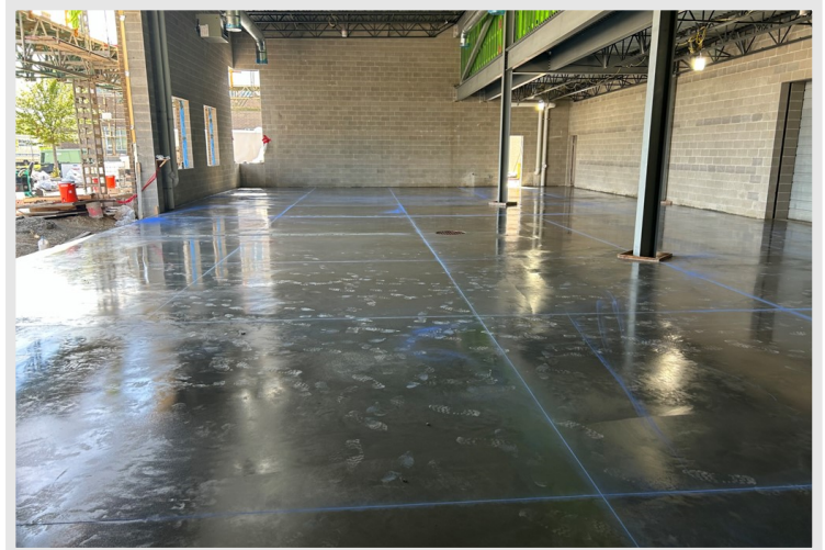
Slab joint layout lines snapped by Findorff concrete crews after the finishing touches were put on the slab floor in the Skills Lab Addition.
