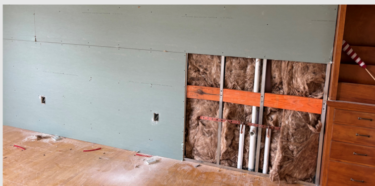
This image is a great showcase of the metal stud framing, plumbing, blocking, and drywall that fits inside the finished wall.
