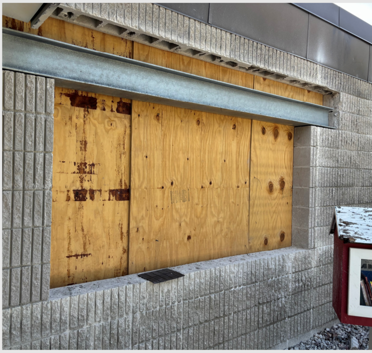
New window openings with the steel lintel in place.
