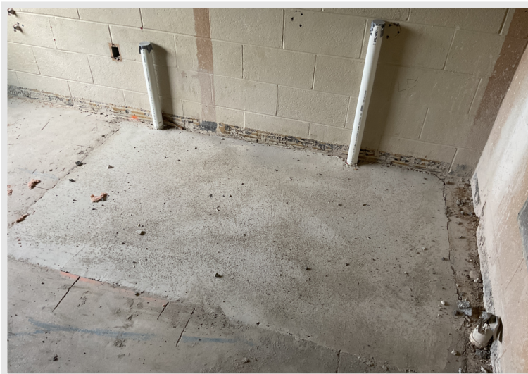
One of the few new concrete infills.
