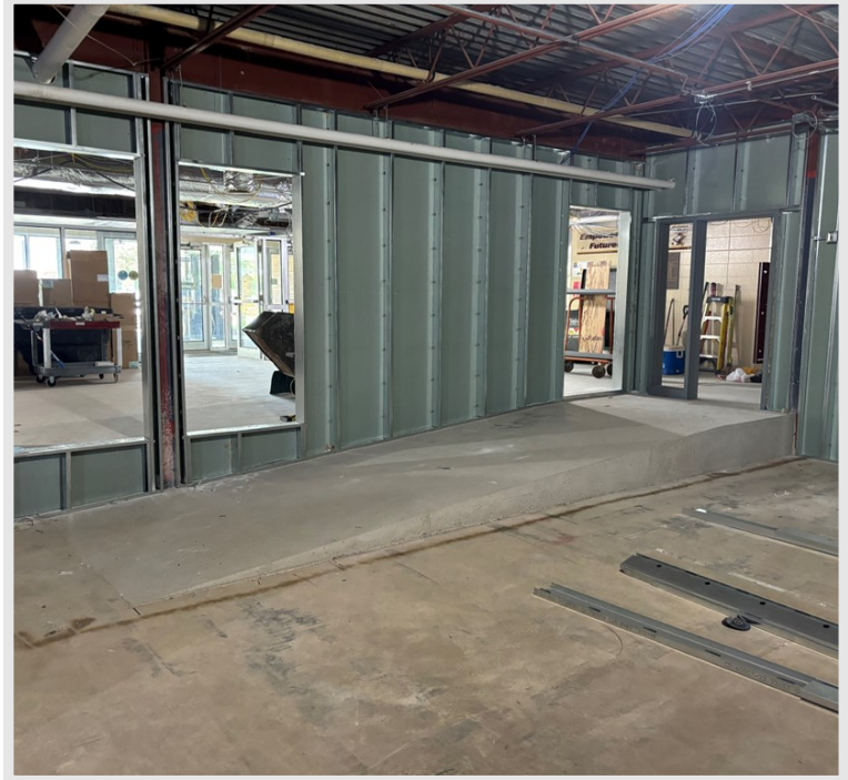
Metal stud framing along with the he freshly poured ramp in the library complies with ADA codes.
