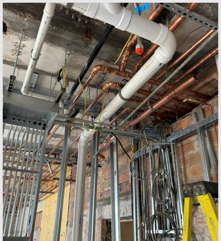
MEP system rough-ins in the main office. Looking Good!
