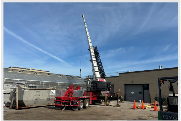
Mechanical crews working to set the final rooftop mechanical units that will serve future classroom and shop spaces.
